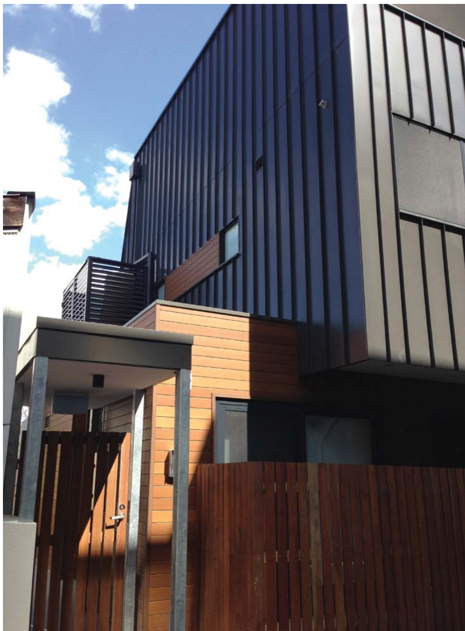
Richmond Veterans Accommodation Project
